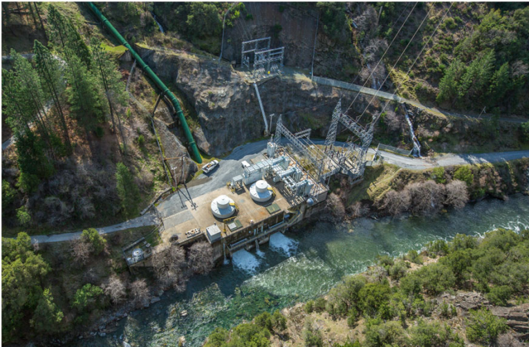
Middle Fork Powerhouse
