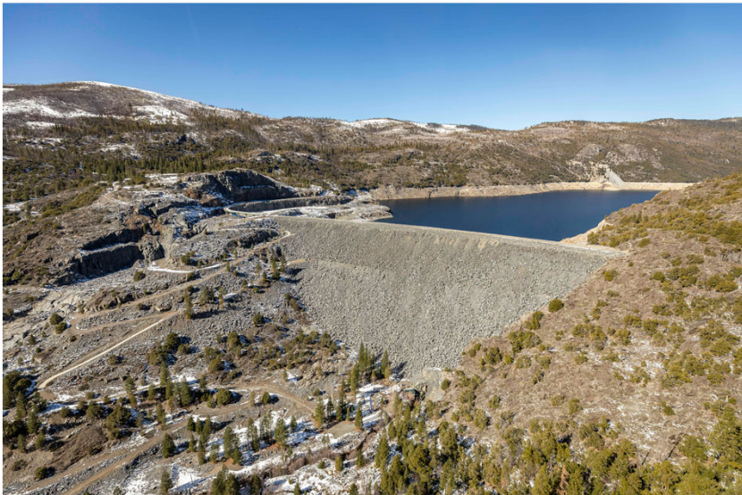
Hell Hole Dam and Powerhouse
