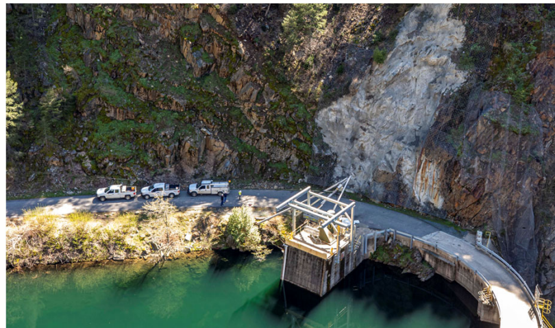
Jib Crane Replacement
