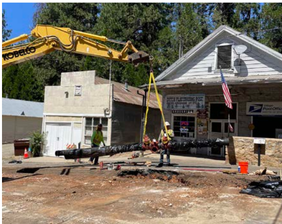
Installation of treated water pipe and a fire hydrant along Main Street
